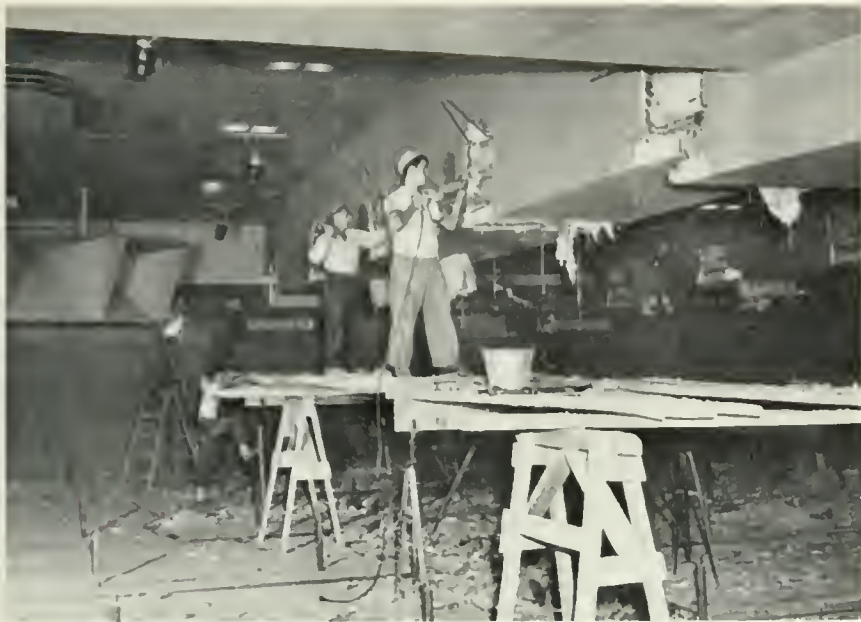
IN REVAMPING NBC'S FAMOUS CONCERT STUDIO 8-H, WORKMEN REMOVE CEILING BEAMS TO MAKE WAY FOR A STEEL OVERHEAD CONSTRUCTION.
