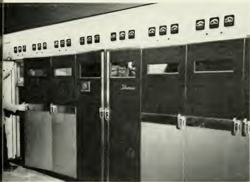
TELEVISION TRANSMITTER OF KRON-TV WHICH COMBINES WITH MODERN ANTENNA TO RADIATE PICTURE SIGNAL TO VIEWERS IN BAY CITIES.
