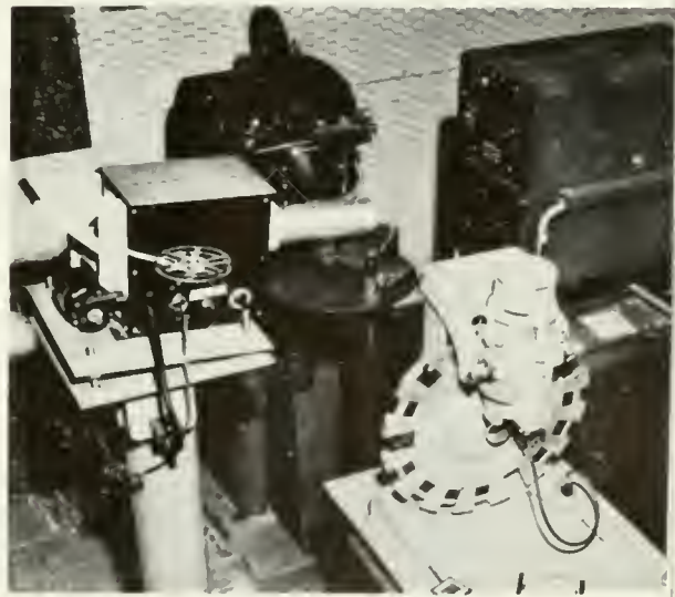
FILM ROOM OF TELEVISION STATION KRON-TV SHOWING PROJECTORS FOR FILMS (REAR), OPAQUE SLIDES (LEFT) AND TRANSPARENCIES (CENTER). CAMERA IS AT EXTREME RIGHT.
